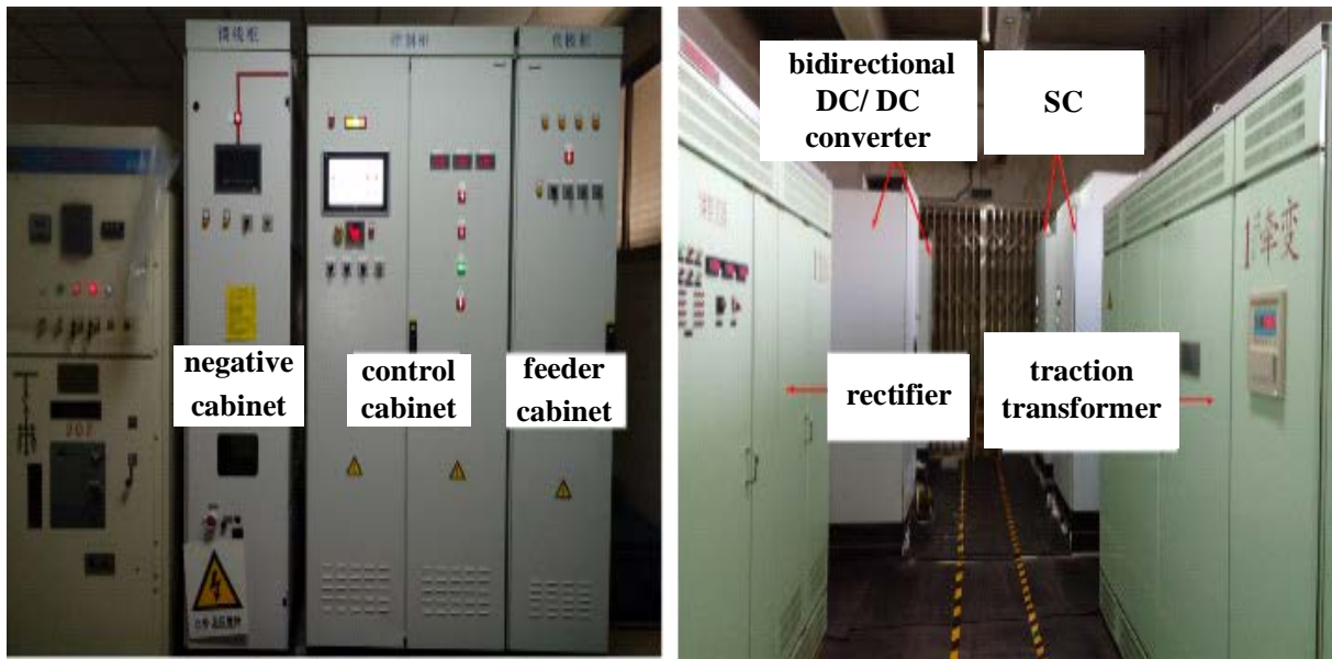
Fig.1 Application of power-type and energy-type hybrid systems
